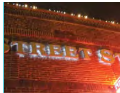
HALO LIGHTING CAN BE AN ELEGANT AND EFFECTIVE METHOD FOR LIGHTING SIGNAGE, ESPECIALLY ON MASONRY WALLS.
