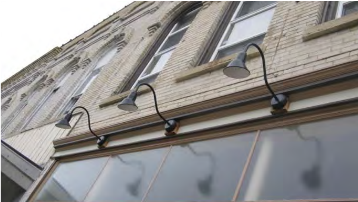
GOOSENECK LIGHTING SUCH AS THIS IS AN ELEGANT WAY TO PROVIDE LIGHTING FOR SIGNAGE OR TO HIGHLIGHT THE BUILDING ITSELF
