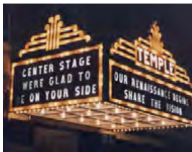
THEATER MARQUEES SHOULD BE RESTORED AND RE-LIT WHENEVER POSSIBLE. HOWEVER, MOVING, FLASHING OR STROBE LIGHTING SHOULD BE AVOIDED IN MOST CASES.
